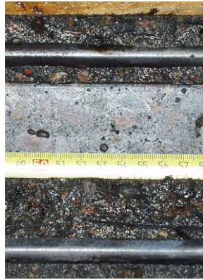
Rebars 2 & 1 Corrosion at 61, 74 cm
