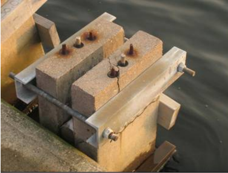
Figure 11 – Intentional cracks in the slabs at the Kristiansand field site.
