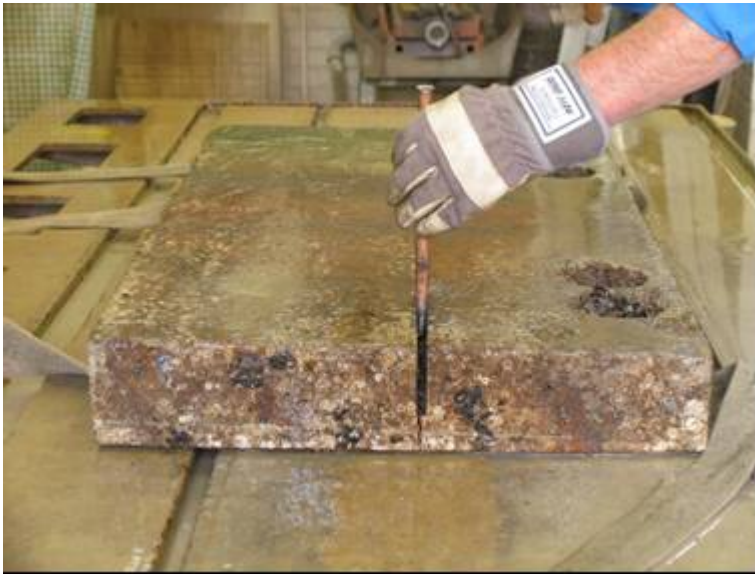
Figure 6 – Release of steel bars for visual examination.
